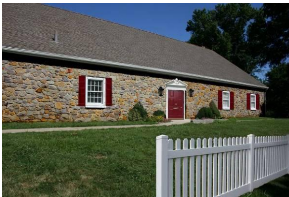
This digitally altered photo shows that a red door with a carved lintel could highlight the entrance. Shutters and stained stone would match other park buildings.
