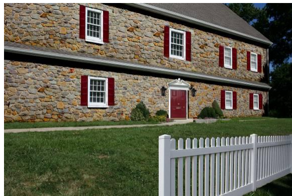
This digitally altered photo shows how a second story could be added to the museum, thus greatly increasing display space while keeping a historic-style facade.
