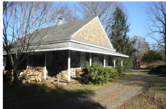
In 1777, Bradford Friends Meetinghouse was place of worship and general community center for the Village of Marshallton.
