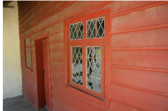
This widow from the Gilpin House gives visitors insights into the challenges of life in colonial time, when large panes of glass were expensive.
