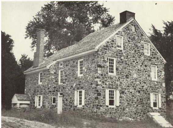
This circa 1952 photo shows the newly reconstructed Ring House which was built on the foundation of the original house that burned down in 1931. 10
